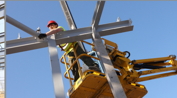
SITE DEMOLITION, ERECTION & CONSTRUCTION
