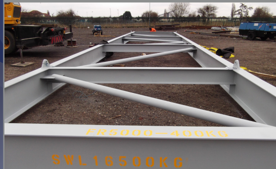
STEELWORK (PAUs PARs Skids)
