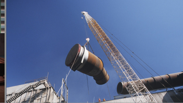
SITE DEMOLITION / ERECTION
