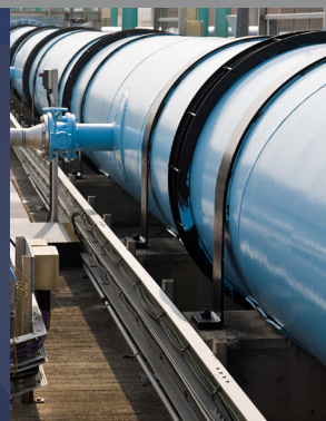
LONDON SEWAGE UPGRADE - THAMES WATER
