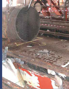
ROUGH RECOVERY - CENTRICA
